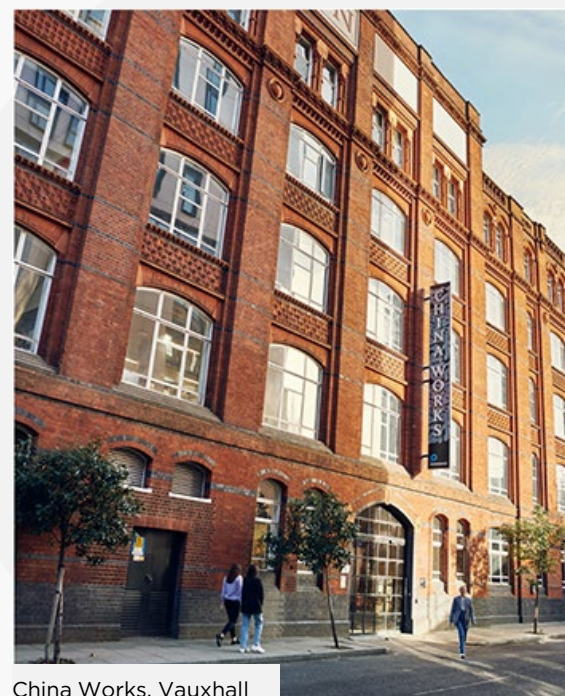
China Works, Vauxhall
